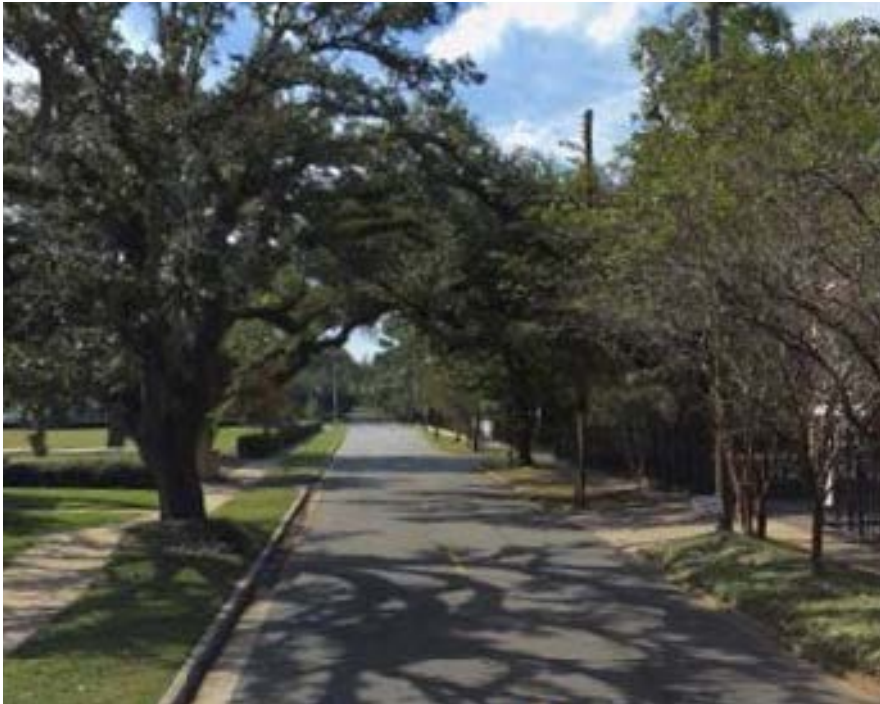
Minor Arterial Typical avenue in Mobile.
