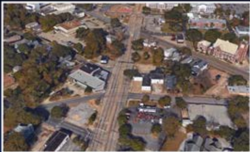
Existing Dauphin St & Springhill Ave Intersection
