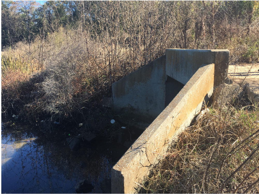
Outfall at Three Mile Creek
