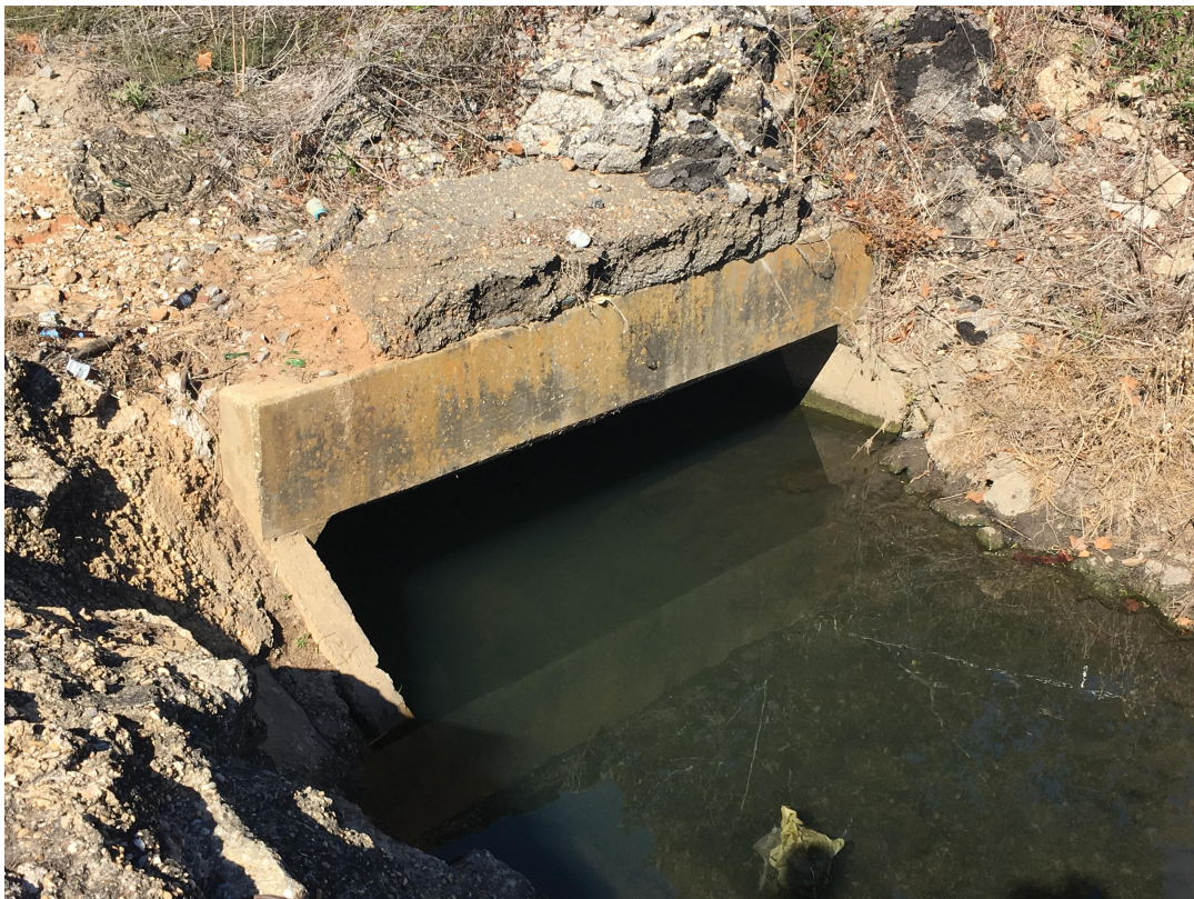
Outfall east of Washington Ave.
