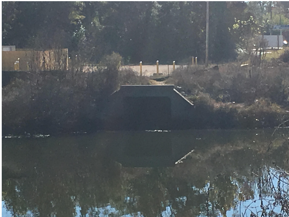
Outfall at Three Mile Creek (looking from the north side)
