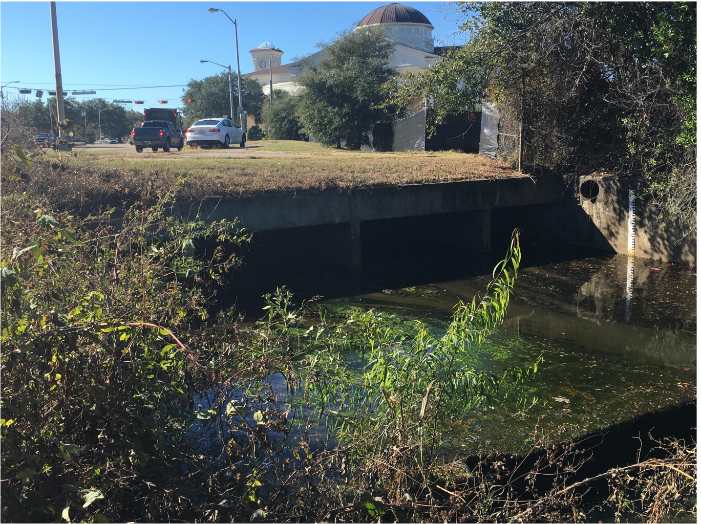
Outfall at One Mile Creek
