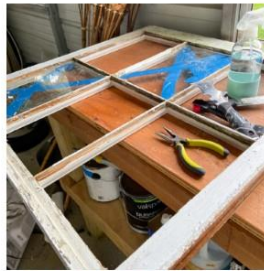
Window sash in process of removing old glazing putty and glass panes
