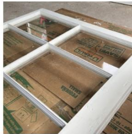
Window sash primed and painted after allowing putty to fully cure
