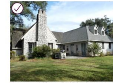
Place an addition so that it is subordinate to the historic residential structure by having a break in the wall plane, and stepping back the addition from the primary facade.
