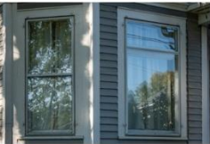
These storm windows have been customized with muntins that match the respective windows, a two-over-two double-hung sash on the left and a fixed picture window with unequal light sizes on the right.
