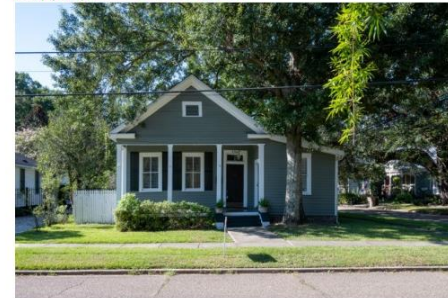
Side additions should be recessed behind the front wall plane of the original structure. This addition obscures the front porch of this contributing residence.
