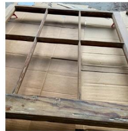
Wood window sash after paint removal
