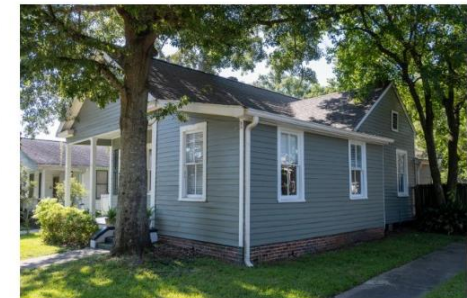
Side additions should be recessed behind the front wall plane of the original structure. This addition obscures the front porch of this contributing residence.
