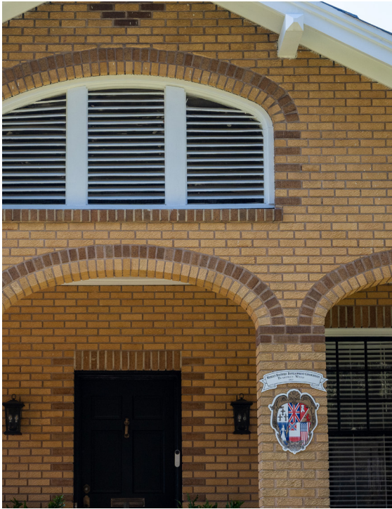
Two-tone brickwork is a character-defining feature of many contributing buildings in Mobile's local historic districts, such as this Craftsman style bungalow in Old Dauphin Way.
