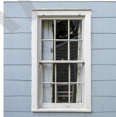
Fully restored window sash reinstalled in framed opening
