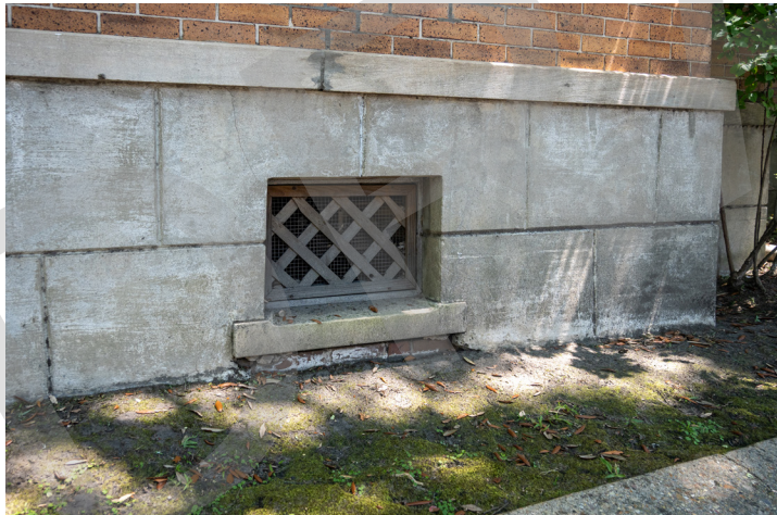
This continuous masonry foundation in Church Street East features decorative iron vent grilles.
