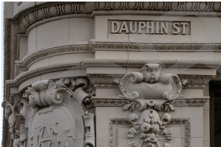
Molded and glazed terra cotta ornamentation in Lower Dauphin
