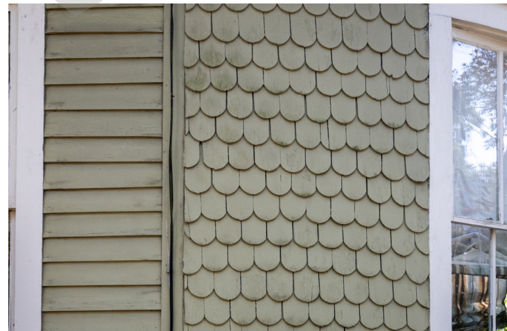
Wood lap and shingle siding in Oakleigh Garden
