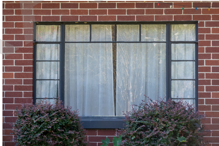
Steel picture and casement window in Old Dauphin Way
