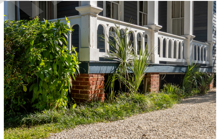
Masonry pier foundations may be left open with no infill between piers, as is seen in this 19th-Century cottage in Old Dauphin Way.
