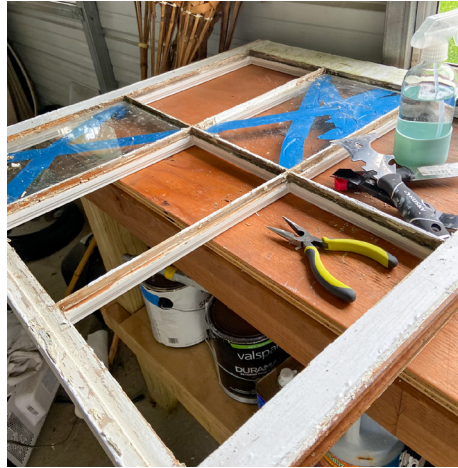
Window sash in process of removing old glazing putty and glass panes
