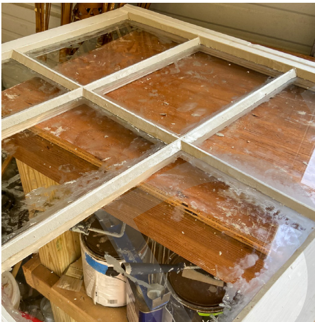
Window sash after application of paint primer followed by reinstallation of glass panes with new glazing points and putty
