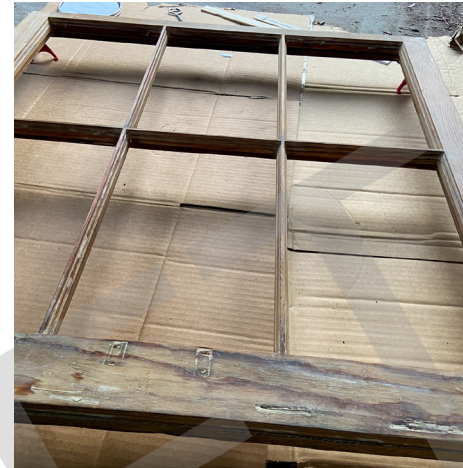
Wood window sash after paint removal
