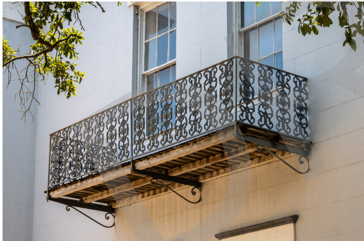
Ironwork balcony in Church Street East
