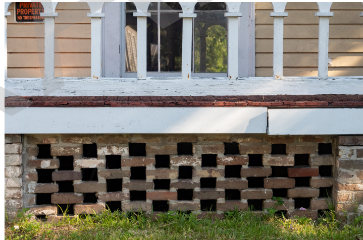
Brickwork lattice is an appropriate infill between masonry piers.
