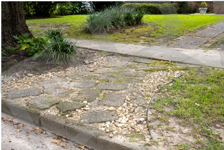
These footpaths in Ashland Place employ a mix of gravel, flagstones, poured concrete, and brick pavers.
