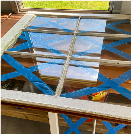
Deteriorated wood window sash removed from framed opening in preparation for repair and restoration
