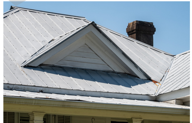
5-V Crimp metal roof in Oakleigh Garden
