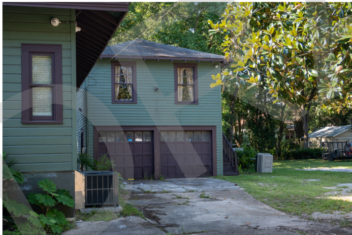
Detached garage apartment in Old Dauphin Way
