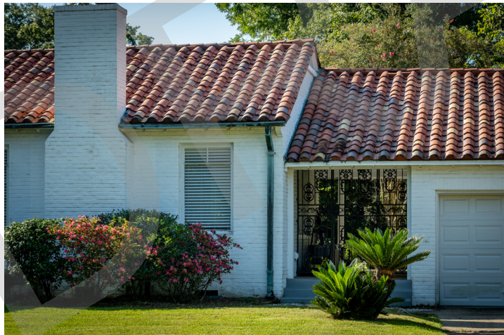
Clay tile roof in Old Dauphin Way
