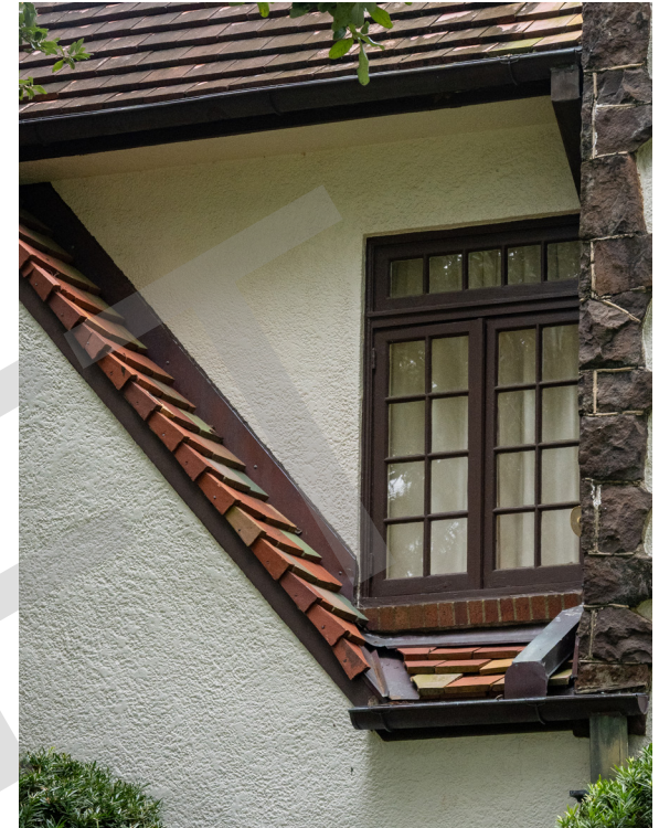
Roof with matching replacement tiles in Ashland Place
