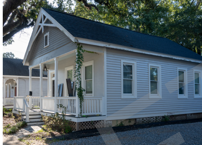
1055 Dauphin after the porch reconstruction.
