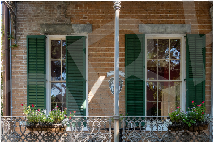
These shutters in De Tonti Square are operable and appropriately sized to fit the window opening.
