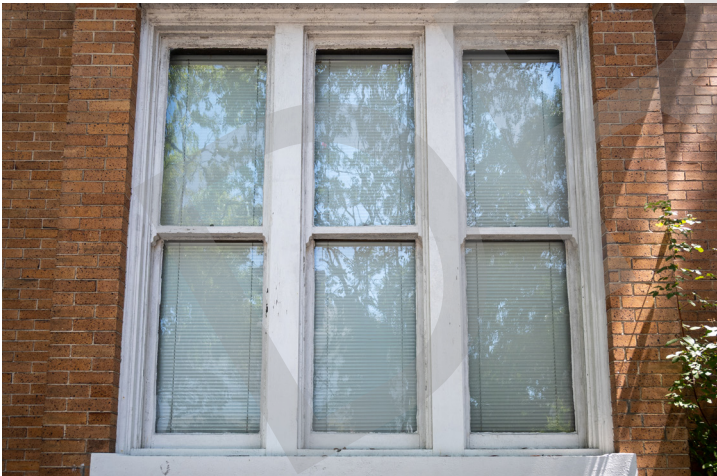
Tripartite window grouping in Church Street East
